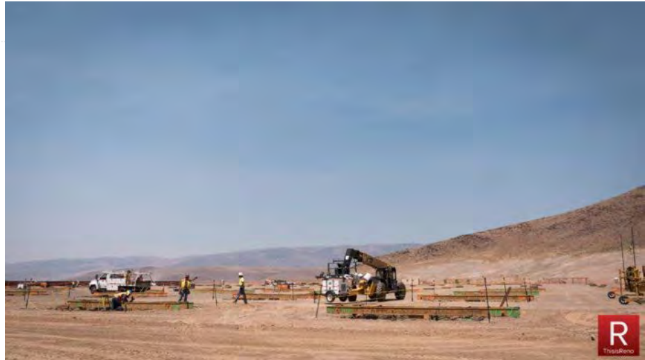
Tesla Gigafactory construction in 2016. Image: Bob Conrad.
