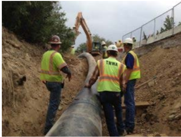
TMWA Workers Install a Water Main Pipeline.
